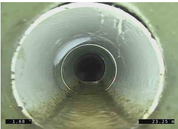
3, 00:04:02, 23.25m (8.81m) Material change / CIPP to PVC
