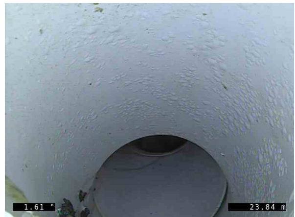
4, 00:04:22, 23.84m (8.22m) The lateral is open, at 10 o'clock / 100mm
