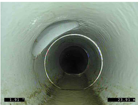
5, 00:04:22, 23.84m (8.22m) The lateral is open, at 10 o'clock / 100mm
