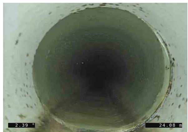
6, 00:04:41, 24.08m (7.98m) Material change / PVC to CIPP
